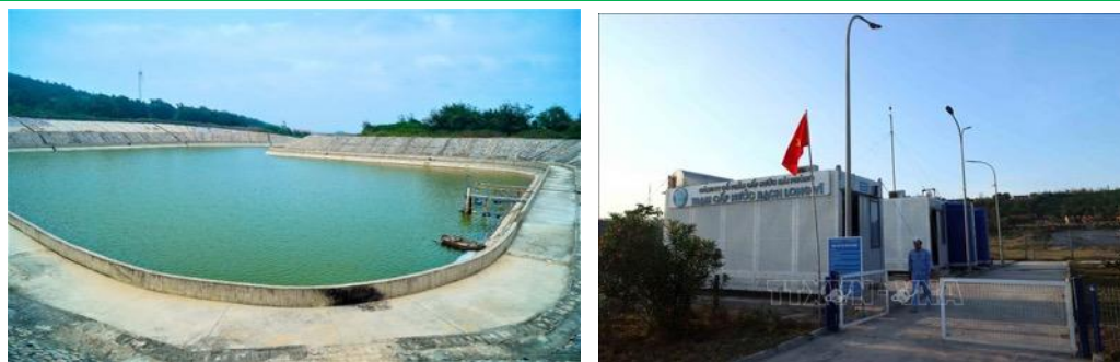
Figure 2.19. Freshwater reservoir with a capacity of 45,000 m 3 and the water supply plant for the residents of Bach Long Vi Island with a capacity of 15m 3 /hour.
