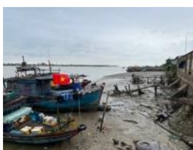
Existing port wharf.
