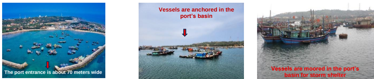
Figure 4.3. Bach Long Vi Port receives approximately 100 vessel arrivals and departures daily.
