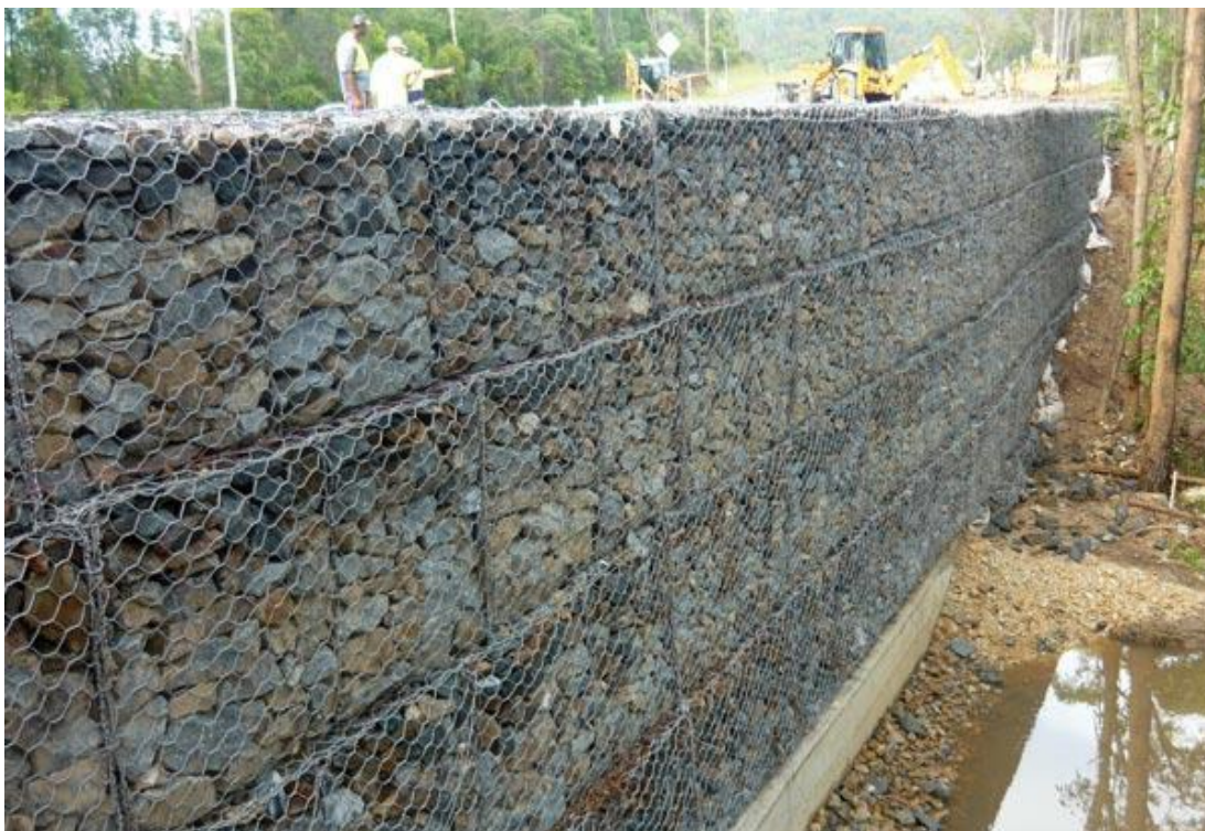
Form. The retaining wall made of supported gabion boxes
