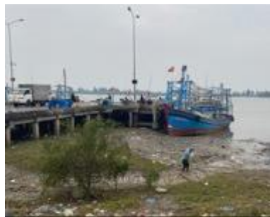
Existing port docks
