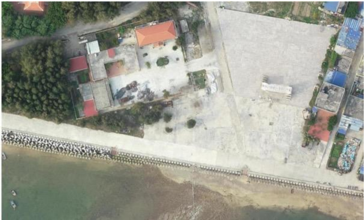
Figure 1.27. Existing status of the service area behind the port
